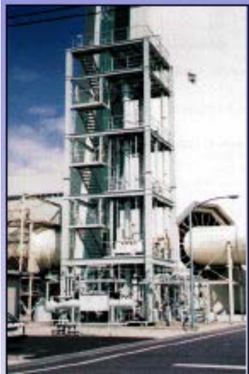
Nanko Pilot Plant (2t/d)
