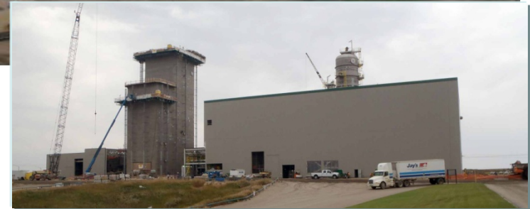
Boundary Dam – Under Construction
